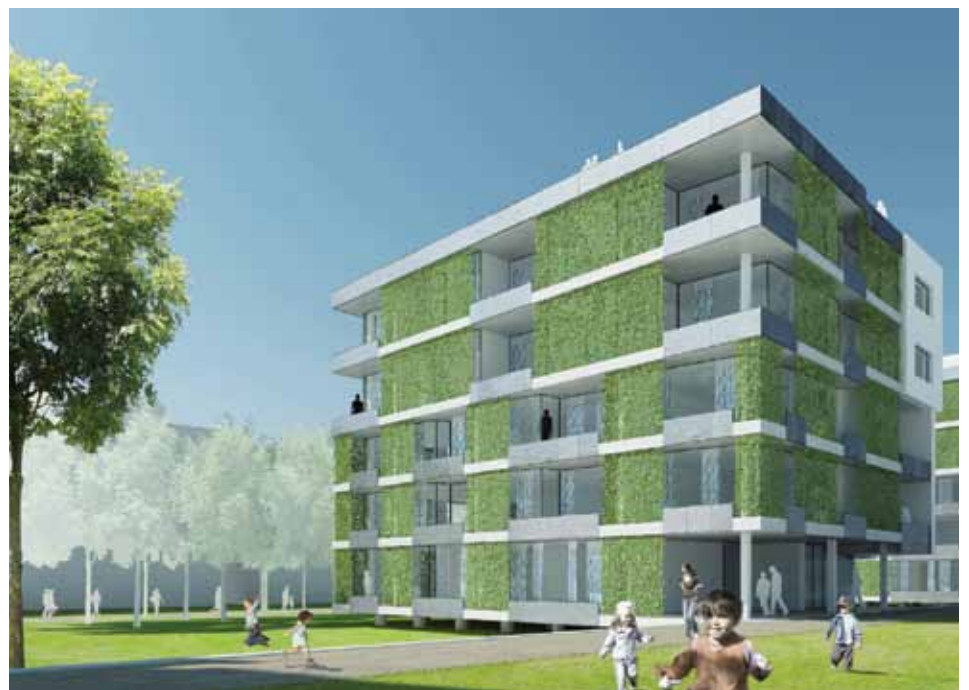
A team of architects from Graz, Austria, has designed a building whose facade contains living algae that can be dried and used in a biogas plant.
